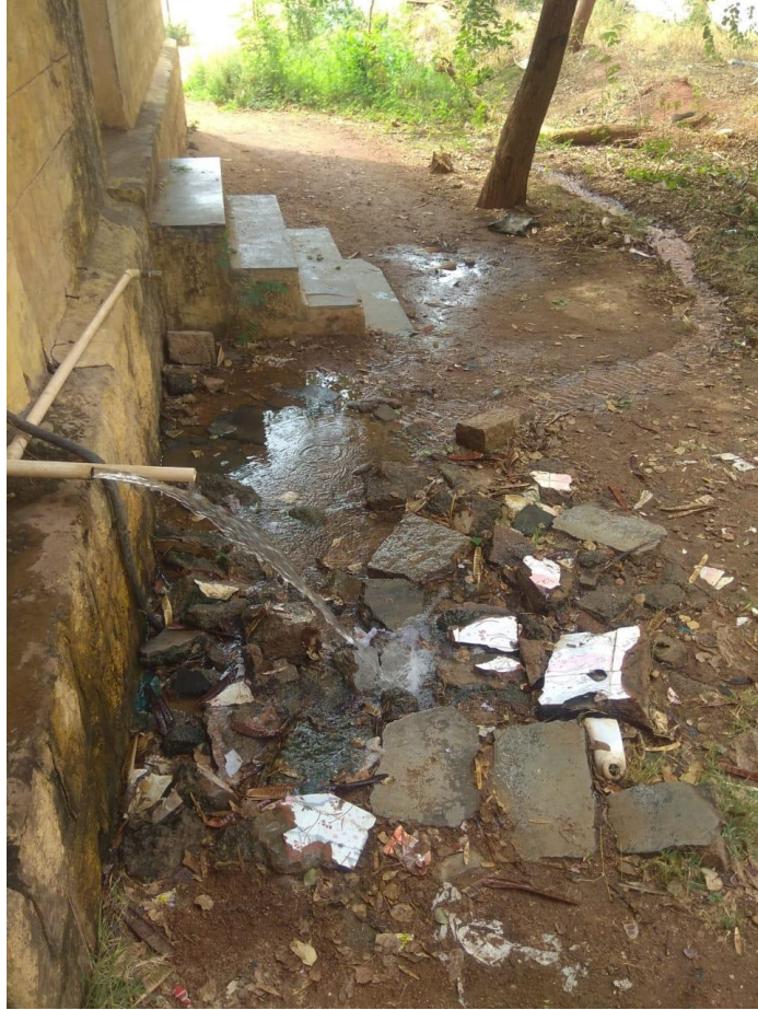
Waste water generated by RO Plant is being channelized to plantations
